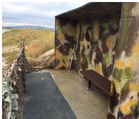
ADA accessible hunt blind was finished by our maintenance/facilities volunteers.
